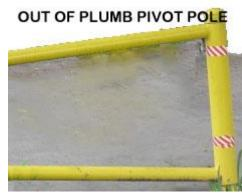
In general, the unsecured condition of these swinging gates has existed due to intentional abuse and vandalism, design and fabrication defects or deferred conditions due to lack of maintenance and repair.
