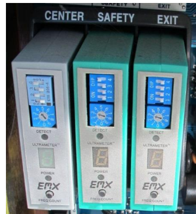
This view of the electronics in a typical gate operator (right) shows three installed modules that are attached to the in-ground loops.
