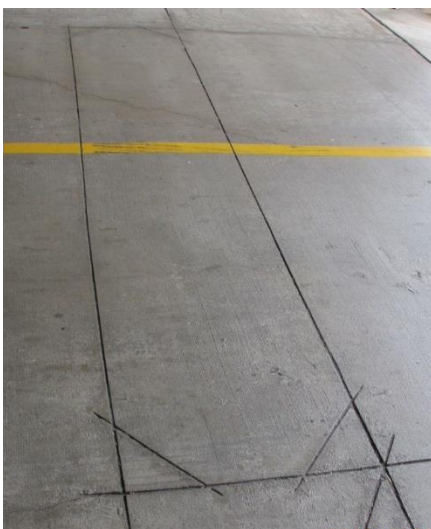
The actual wire ground loop installed in this driveway (left) is not visible. The saw cuts indicate that a small trench has been made to place the ground loop wire. Typically, the clipped or rounded corners and trail show the position of the loop. In many cases, additional loops have been installed due to improper original placement of the in-ground loop. It is important to verify which of the trenched ground loops are currently connected to the motor controller.
