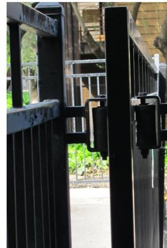
There are usually at least two components that are observed to be missing or defective regarding gate stops. One is the absence of any restricting stop component, the other are missing or broken pinch rollers that are used to guide and align the sliding gate as it opens and closes.
