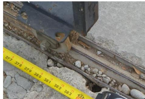
checked for full attachment to the pavement where it is positioned. Whether it is recessed or surface mounted, the entire length of the track must be constantly checked for any materials that would cause a derailment. These obstructions can include rocks, pebbles, trash, or other debris that can affect the connection between the roller and track.
