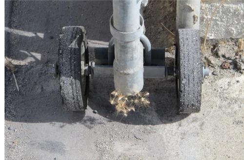
These rolling wheels take a portion of the sliding gate weight and need to be properly maintained for alignment so that the gate travels in a straight line.
